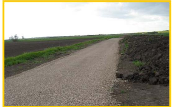
(ii) Braes of Doune Windfarm, near Stirling: In excess of 20km of 5.5m wide access roads had to be constructed over peaty silty clay conditions to allow the construction of, and future access to 36 wind turbines. Constructed using graded granular fill and crushed rock, the E'Grid biaxially reinforced roads (some floating) ensured smooth access over
