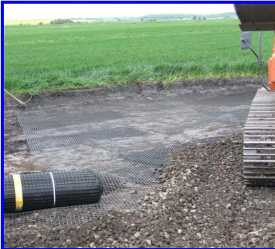
(i) Fenlands 'Red Tile' Windfarm, Huntingdon: a design proposal was offered to the Contractor highlighting how reinforcing the unpaved road with E'Grid 3030 could reduce the required sub-base thickness and save on both excavation and imported materials. Based on anticipated traffic loadings and the actual subgrade soil strength an unreinforced sub-base thickness of 603mm was required. By including a layer of E'Grid 3030 at the sub-
