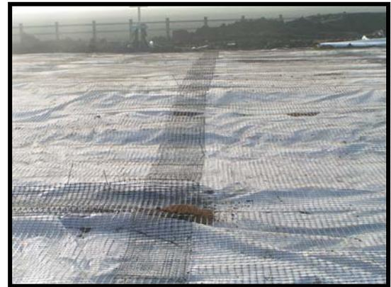
In order to provide continuous strength in the main load carrying direction E'Grid 3030 was installed across the width of the carriageway. Product continuity along the length of the carriageway was provided via a 300mm overlap, secured during the construction phase with plastic cable ties.
